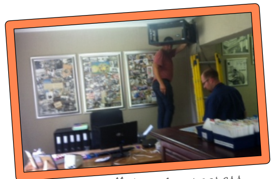
IT installation in progress
